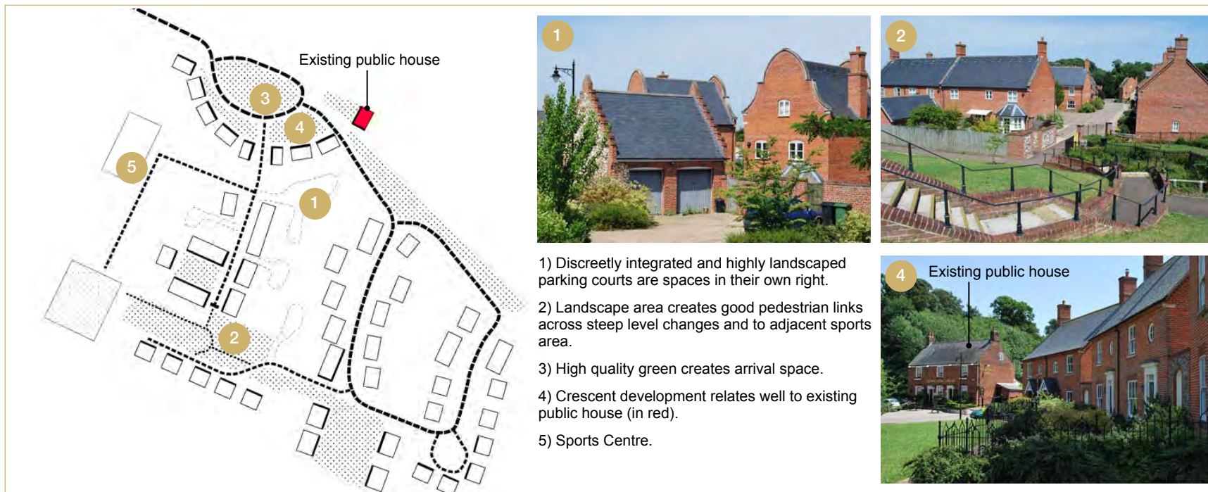
Figure 4.12: Trowse, Norfolk, a housing development that creates a strong sense of place
