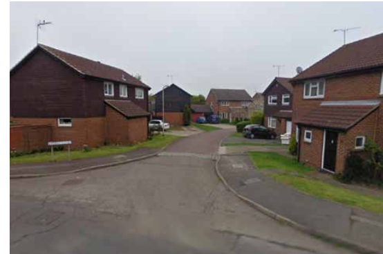
Figure 3B.24: Clusters of houses that look inwards towards each other rather than defining a street in Woosehill
