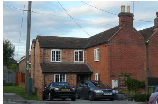
This example demonstrates an example of an extension with a ridge height that is subordinate to that of the original property
