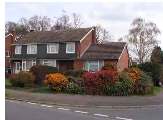
Figure 4.36: Extensions that relate well to the original buildings
