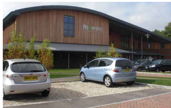
Figure 7.10: The use of materials, the canopy and overhang of the roof help to create a human scale for this community centre
