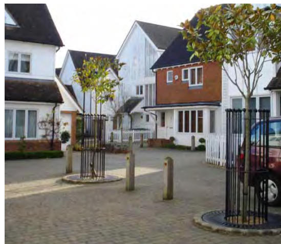
Figure 5.6: Cul-de-sac or mews streets can be designed as positive spaces by thinking about the space as somewhere for other activities as well as just functional requirements such as parking and turning circles
