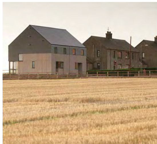
Figure 8.8: New development can respond to existing rural development by using a similar massing and form, without being designed as a pastiche
