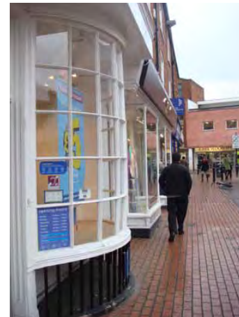
Figure 7.24 Historic features such as curved glazing should be incorporated into new shopfronts as here at Halifax, Wokingham
