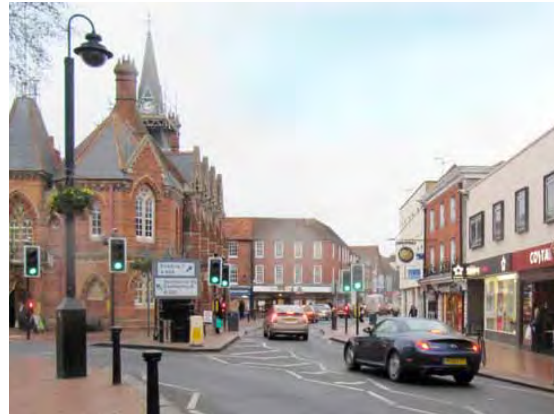
Figure 3B.3: Wokingham Town Centre has an urban centre character; buildings adjoin each other and tightly define the street pattern
