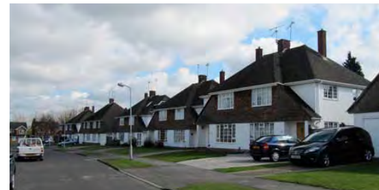
Figure 4.17: Some areas are characterised by open plan front gardens. In this case the set-back from the street provides sufficient privacy for rooms on the frontage to have large windows
