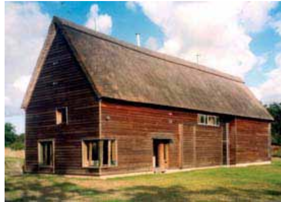
Figure 8.13: In this example a variety of openings have been incorporated to bring light into the interior without being overly domestic in style
