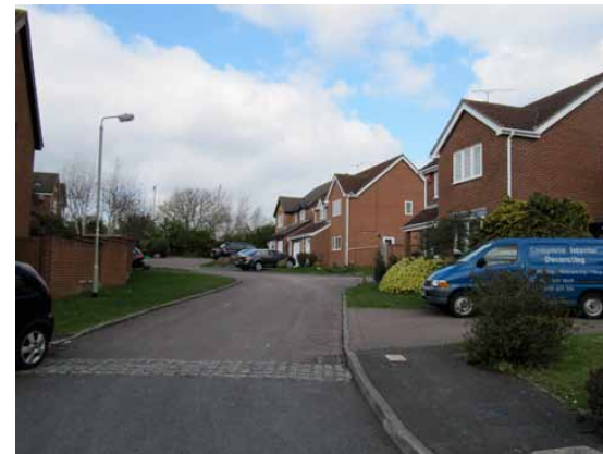
Figure 3B.25: Curved streets and an informal and varied building line in Earley
