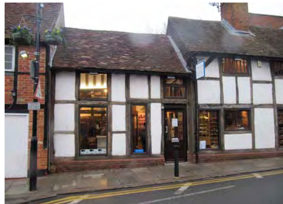
Figure 7.30: In this traditional building a high quality wooden and glass shopfront has been inserted that respects the character of the existing building whilst providing a modern, stylish solution
