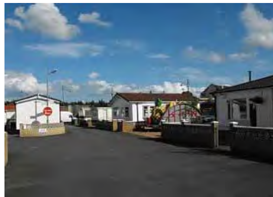
Figure 4.38: An example of a well laid out site
