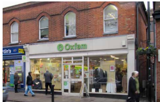
Figure 7.26: Shopfronts should respond to the building as a whole. At Oxfam in Wokingham the symmetry of the shopfront relates to the symmetry of the upper storeys
