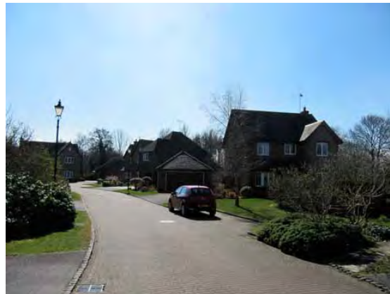
Figure 3B.23: Houses in informal suburbia are detached or semi-detached and grouped in small clusters around shared culs de sac as here in the more suburban areas of Twyford
