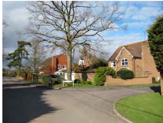
Figure 3B.11: Buildings are loosely arranged and of a variety of character in Spencers Wood
