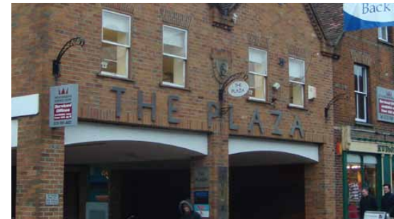
Figure 7.31: Where a building has not been designed with a fascia, individually mounted lettering can be an appropriate solution
