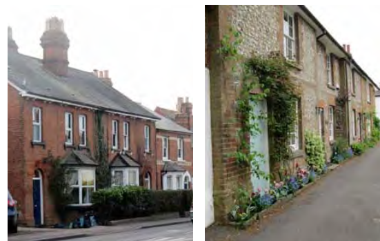
Figure 4.24: Different ways to provide appropriate levels of privacy on street frontages. Victorian houses with large bay windows tend to have a front garden with boundary hedge. Cottages without front gardens have taller, narrow windows to reduce the potential for looking inside
