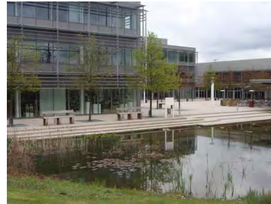
Figure 7.1: In this development, Green Park, an attractive public realm has been created which is well used
