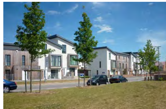
Figure 4.33: Street scenes can be designed so that roofs are at the most suitable angle for efficient solar panels
